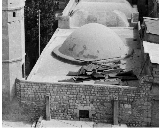
Outside facade of Eastern wall of Prayer hall (Jean-Claude David, 1980)
