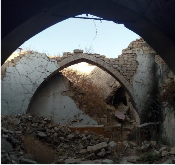
Damaged vault, western the prayer hall Museum for Islamic Art-Berlin, September 2019)
