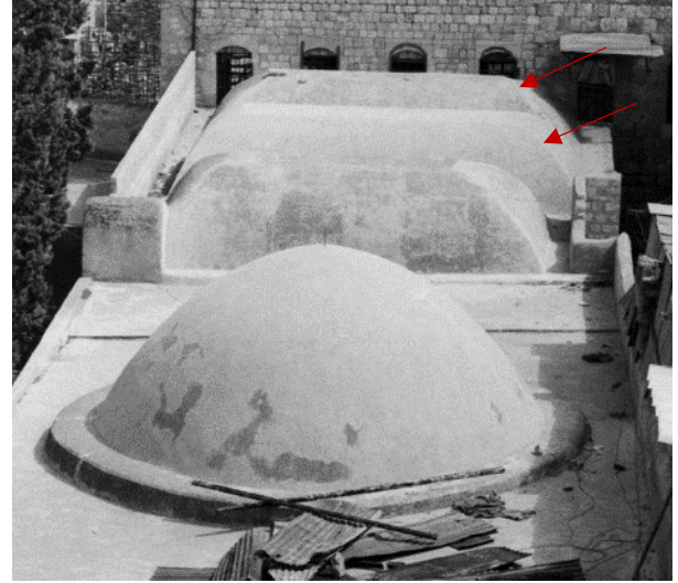
Vaults of Prayer hall ceiling (Jean-Claude David, 1980)
