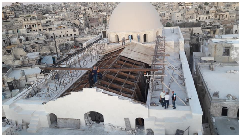
Rebuilding the wooden roof of the Maronite Cathedral, Mohamad Ahmad, September 22, 2019
