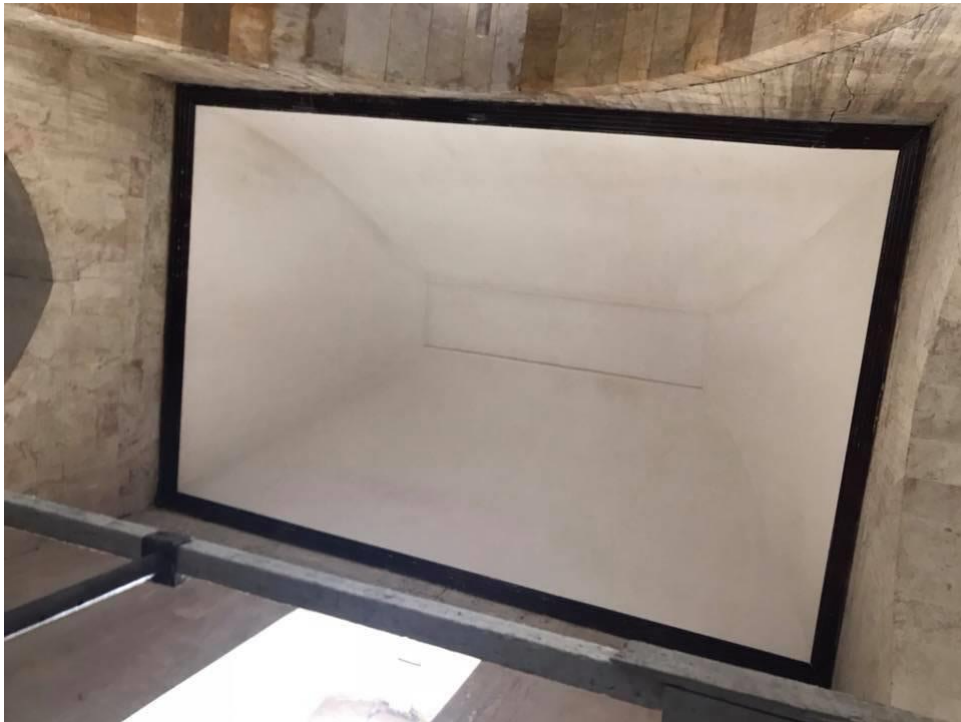
Greek Orthodox Church, the vault after restoration
